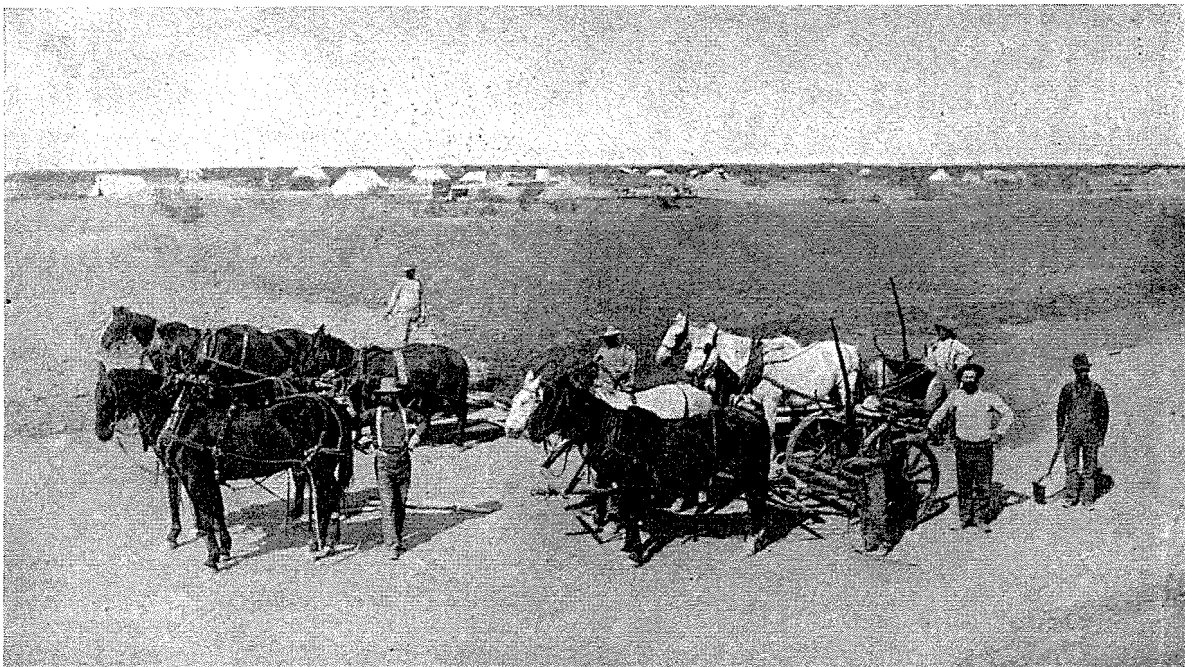
W. W. Masten's Grading Camp in 1901. Dozens of Scraper Outfits like these built the Canals
