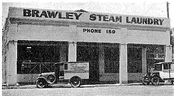
Plant of the Brawley Steam Laundry
