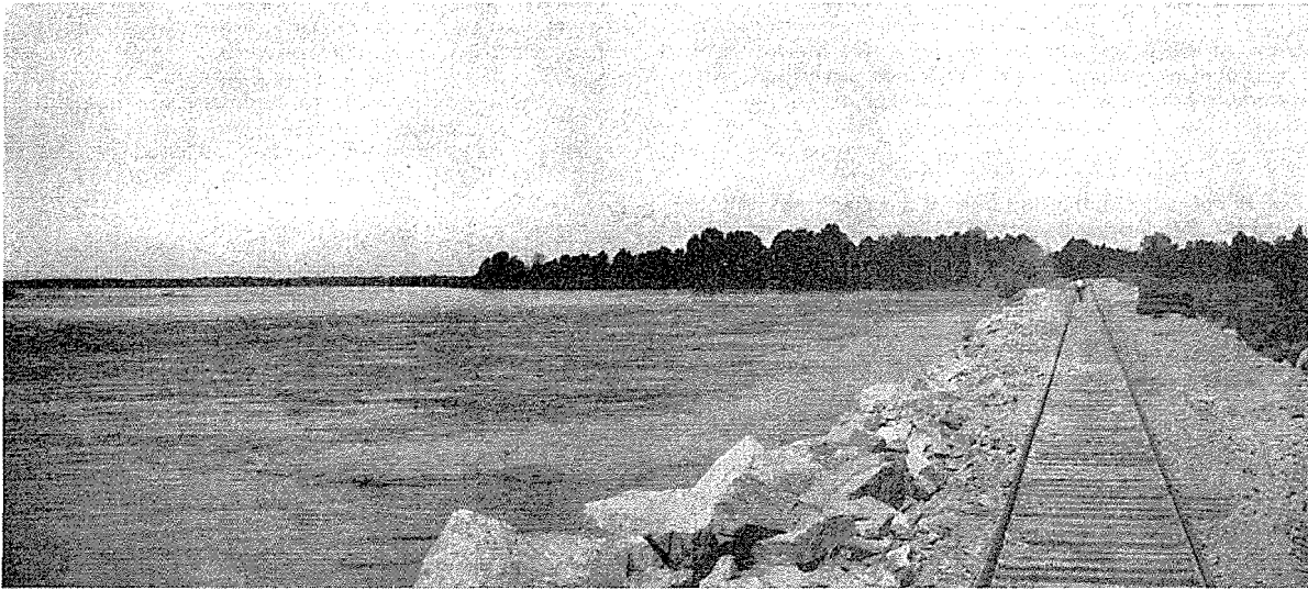
The District Maintains Thirty-one Miles of Rock Faced Levees in Mexico
