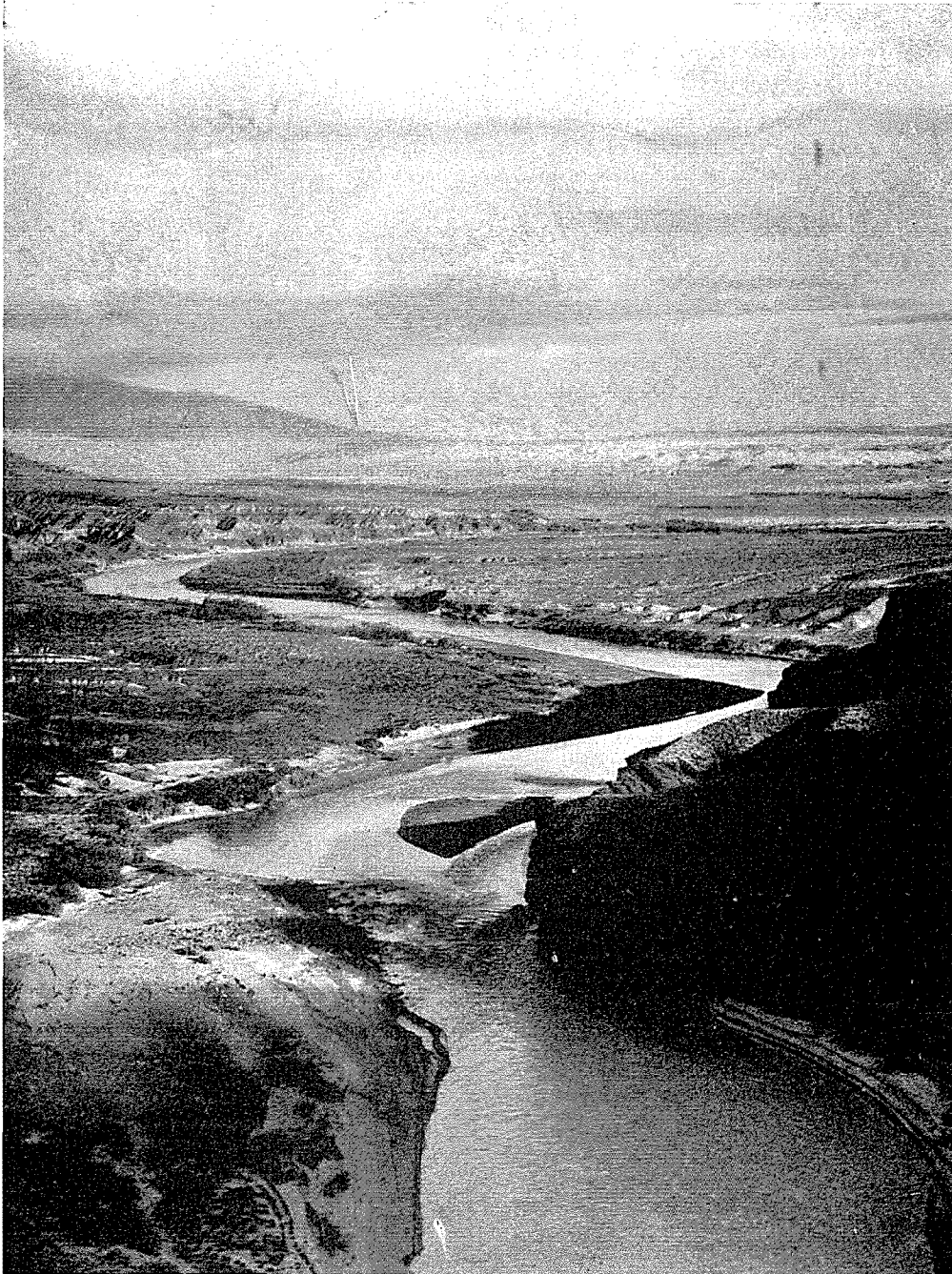
Reservoir Site where 26,000,000 Acre Feet of Water will be Stored Behind Hoover Dam
