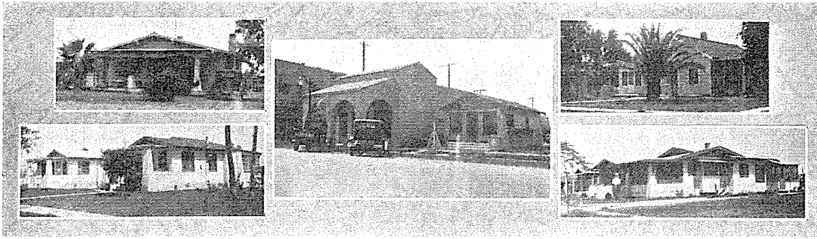
W. I. Stone's Office (center) and Four of the Eighty Homes He has Built in the County Seat
